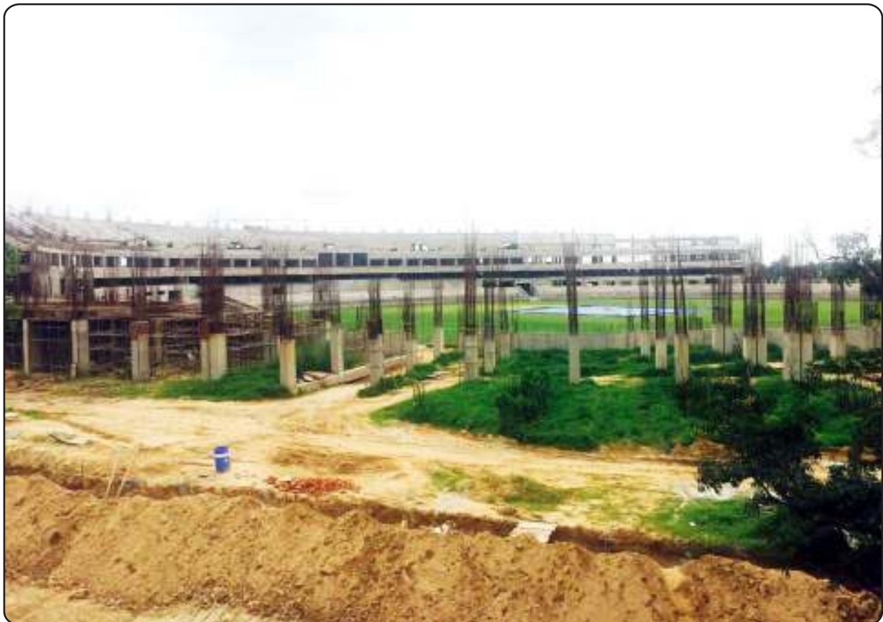
Structural work in progress at the New Stadium
